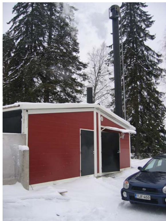
300 kW heating station of Bovallius Foundation, fired with wood chips.
