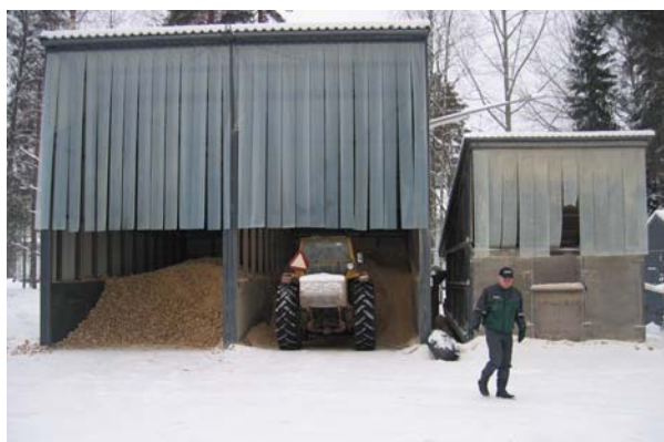
Wood chips storeroom of Nikkarila School of Forestry.
